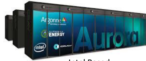
Intel Based (Being installed)
