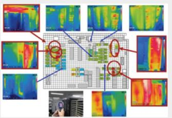
Next, Fujitsu compared the heat generation of equipment in the server room to the air-conditioning capacity. This exercise showed that there was more than enough air conditioning. The conclusion was that it should be possible to reduce power consumption by shutting down one air-conditioning unit.
