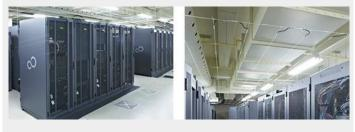
In the Cloud Center, a few optical fibers snake along the ceiling at 50 cm intervals, runs around the fronts and backs of server racks and even under the floor before it connects to the measurement device.
