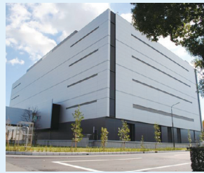
The new annex of Fujitsu's Tatebayashi System Center
