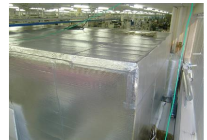
Insulation of burn-in facilities
