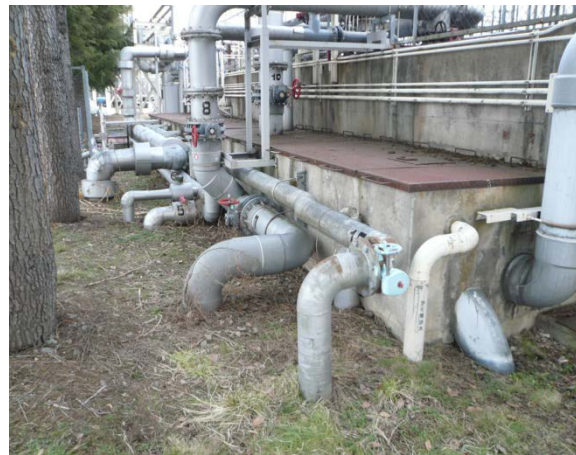
Before moving piping above ground
