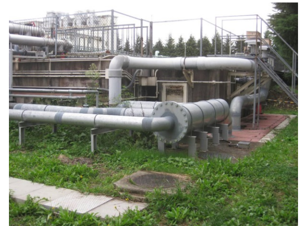
After moving piping above ground
