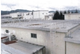
Before roof painting
