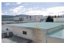
After roof painting
