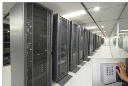
Server room Approx. 300 server and storage units onsite are used to test and demonstrate customer ICT systems
