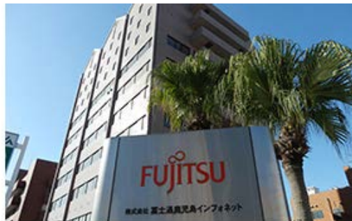
Fujitsu datacenter (Fujitsu Kagoshima Infortnet Limited)
