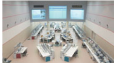
The Integrated Control Room of Tatebayashi System Center
