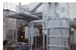
Decompression dehydration dryer (left), membrane concentrator (right)
