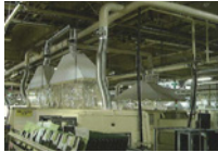
Waste-heat ducts and insulated jackets are used on the reflow furnace.
