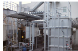
Decompression dehydration dryer (left), membrane concentrator (right)
