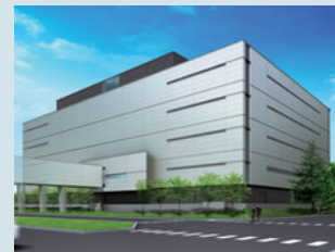
Eco-friendly data center that promotes energy savings from diverse viewpoints.
