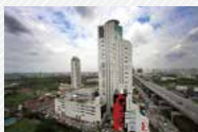
A datacenter in Thailand where Fujitsu has started providing cloud services
