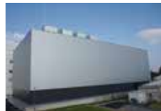
Exterior view of the new Akashi System Center building
