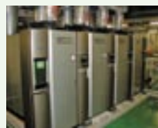
Arai Plant Boiler Installation
