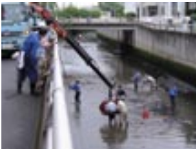
Waste removal project at Sumiyoshi River, Oita City.
