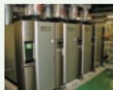
Arai Plant Boiler Installation
