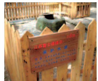
Safety fence made from discarded pallets
