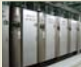
Small boilers burning natural gas
