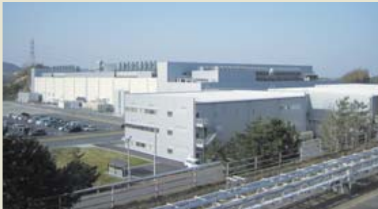
The new wing of the Mie Plant
