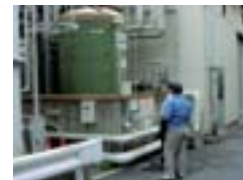
Inspecting chemical tank protection (protecting against leakage)
