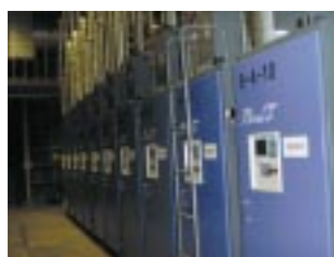
Small through-flow boilers at the Iwate Plant
