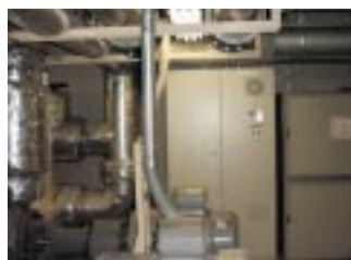
A pump inverter at the Iwate Plant
