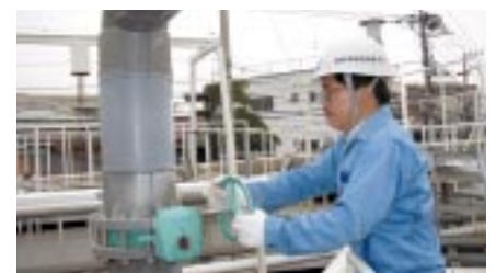
A wastewater disposal facility at the Kawasaki Plant
