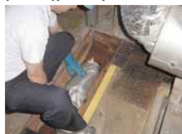
Placement of sandbags along the upper part of a wastewater ditch to prevent drainage into sewers
