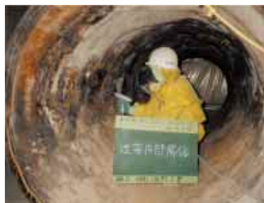
Demolition of an incinerator chimney interior (Fujitsu Numazu Plant)
