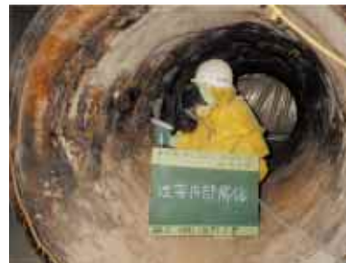
Demolition of an incinerator chimney interior (Fujitsu Numazu Plant)
