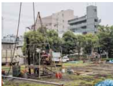
Purification equipment (Fujitsu Kawasaki Plant)
