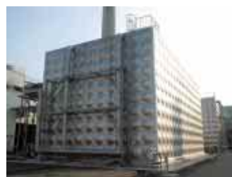
Reservoir as a heat sink (Fujitsu Mie Plant)
