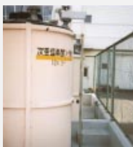
Embankment at waste water treatment facility to contain chemical spills (Kawasaki Plant)
