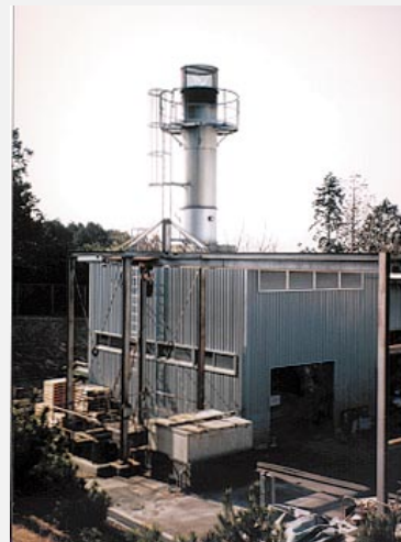
Abolished incinerator (Numazu Plant)
