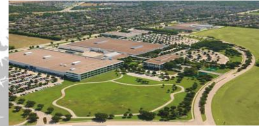
Fujitsu Network Communications, Inc.
