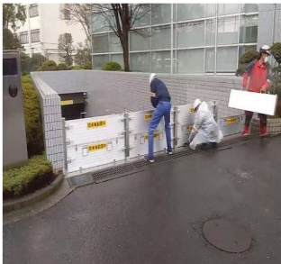
(a) Removable watertight panels
