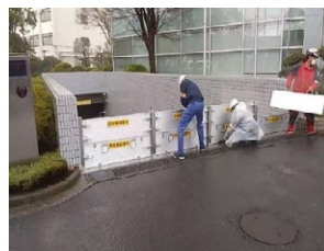
(a) Removable watertight panels
