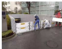
(a) Removable watertight panels
