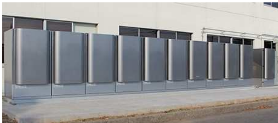
The fuel cell power generation system installed at Fujitsu Frontech's Kumagaya SSC
