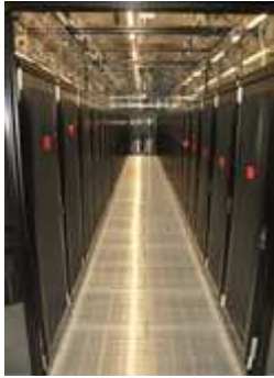
Cold aisle capping and blanking panels Left – Germany Right – UK
