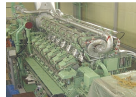
Gas-engine power generator
