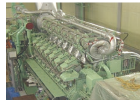
Gas-engine power generator
