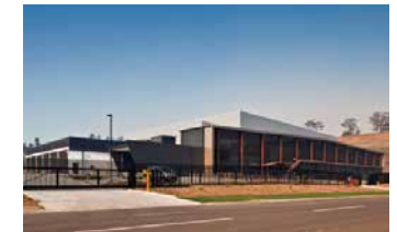
Western Sydney Data Center
