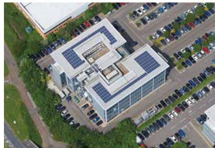
Rooftops with solar panels installed
