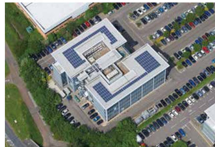
Rooftops with solar panels installed
