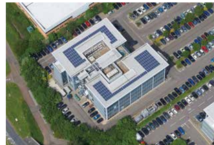
Rooftops with solar panels installed
