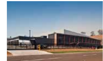
Western Sydney Data Center
