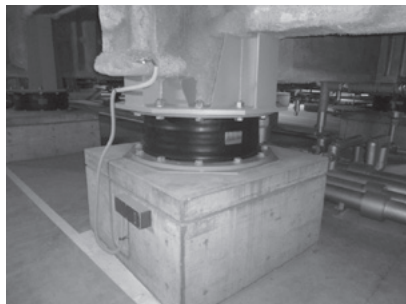
(a) Laminated-rubber seismic isolation device
