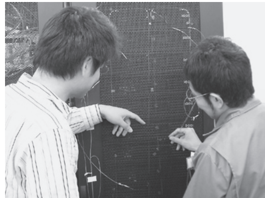
Figure 4 Installation of optical fibers in a server rack.
