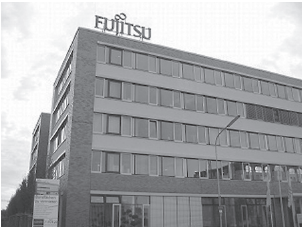
Figure 2 New office building.
