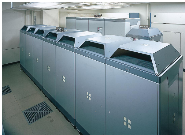
Fig. 1— Supercomputer system VPP300/16R, VX/4R, VX/1R installed in National Astronomical Observatory (NAO), Tokyo, Japan.
