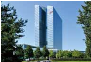
Fujitsu Technology Solutions headquarters in Munich
