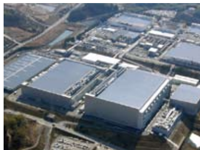
Fujitsu Semiconductor's Mie Plant employs seismic isolation construction
