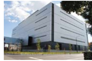
New annex at the Fujitsu Tatebayashi System Center
