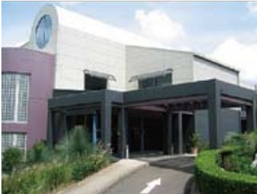
Fujitsu's second datacenter in Sydney has launched public cloud services
