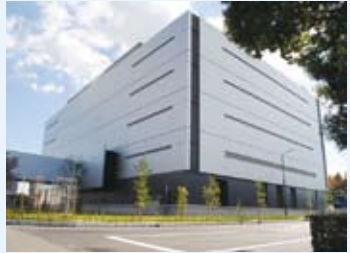
The new annex of Fujitsu's Tatebayashi System Center
