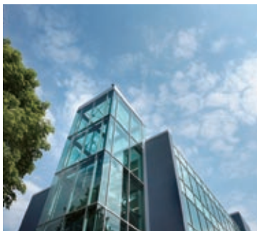
Fujitsu London North Data Centre equipped with cutting-edge technology
