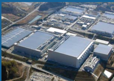
Mie Plant for Advanced Logic LSI Production The Mie Plant produces LSI devices on 300mm wafers. Fab No.1 has been onstream since April 2005, and Fab No. 2, which utilizes 65nm process technology, became operational in April 2007.
