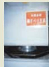
Seismic isolation device (rigid slider support)
