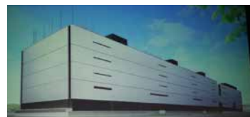
External view of the Tatebayashi Data Center's new annex
