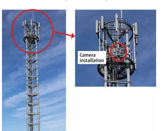
also confirm the damage status of the base stations' communications equipment. Images picked up by the cameras can be assessed in real time, which is expected to aid in the prompt recovery of base stations.
